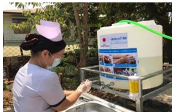
Installing hand-washing stations (UNICEF, Myanmar)
